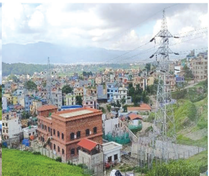
Mulpani Substation and Dense Load Centers
