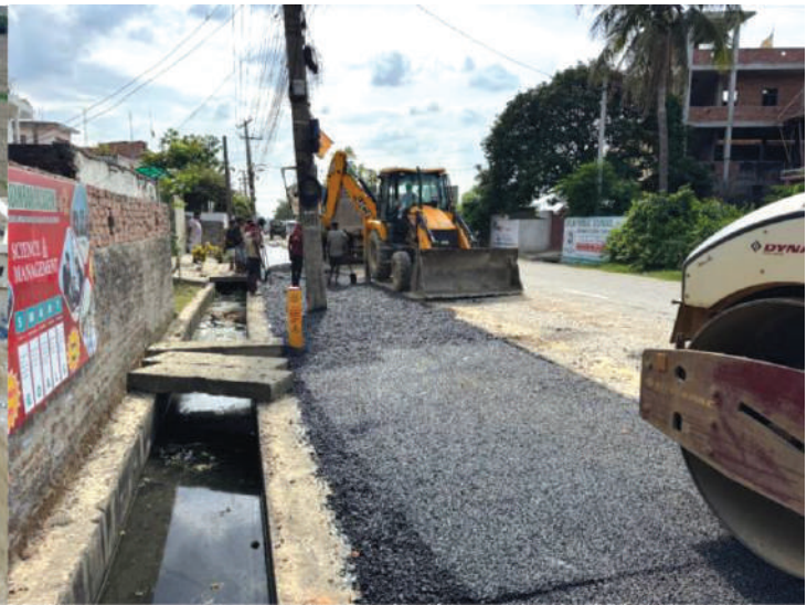
Road Restoration Work at Birgunj
