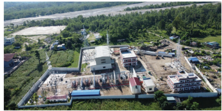
Overall layout of Amlekhgunj Substation
