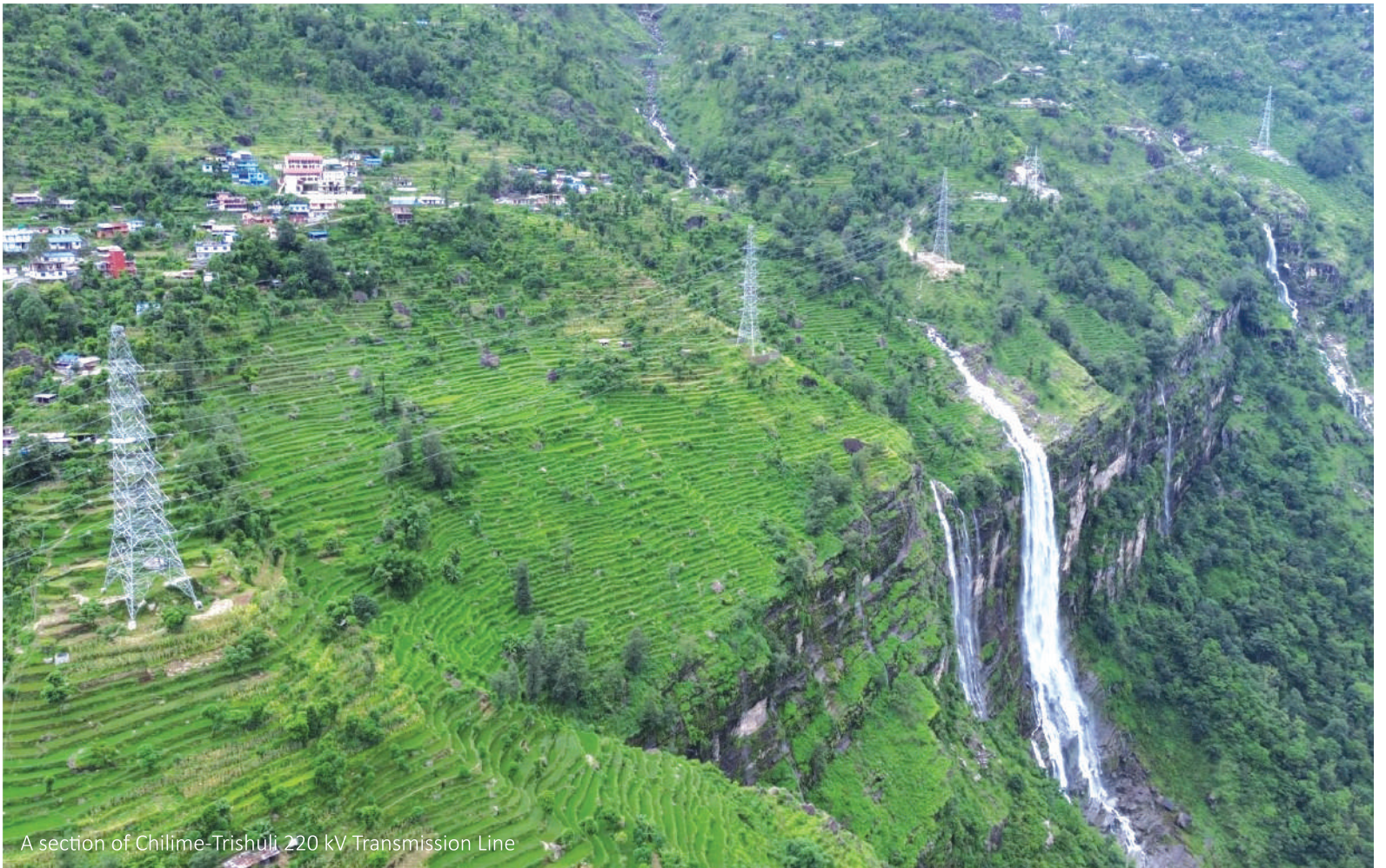
220/132 kV Matatirtha Substation
