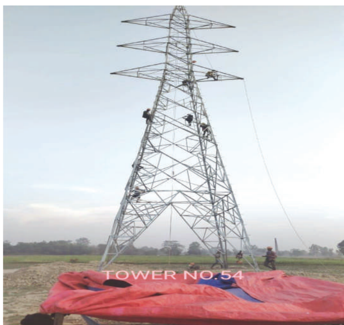
Erection of Tower No. 54
