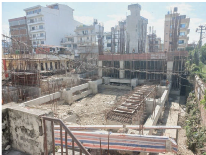
Under Construction Patan Substation
