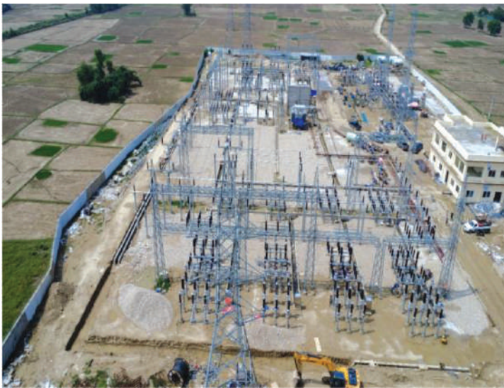
Prasauni Substation under construction
