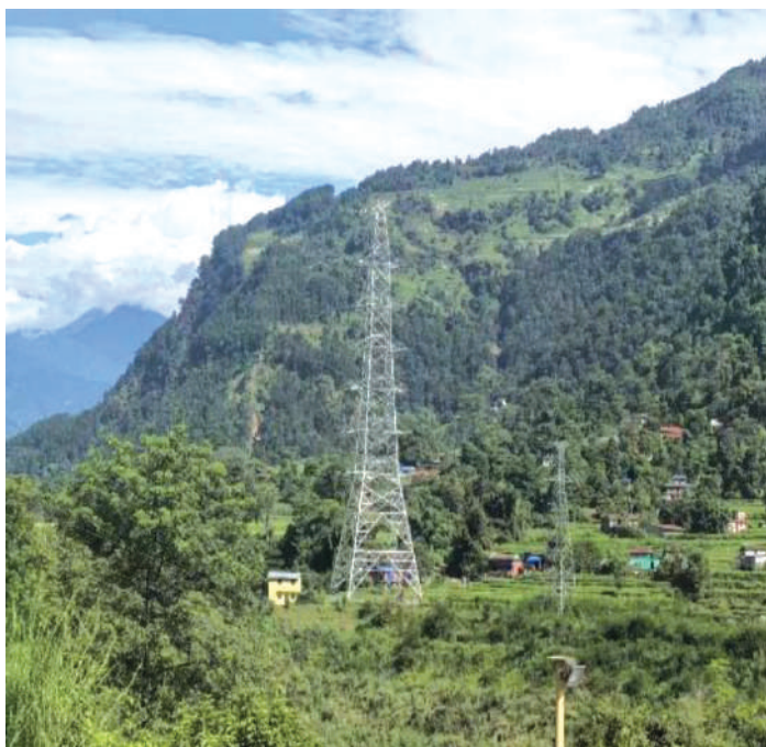
Multi circuit tower erected tower in Khudi Udipur Section
