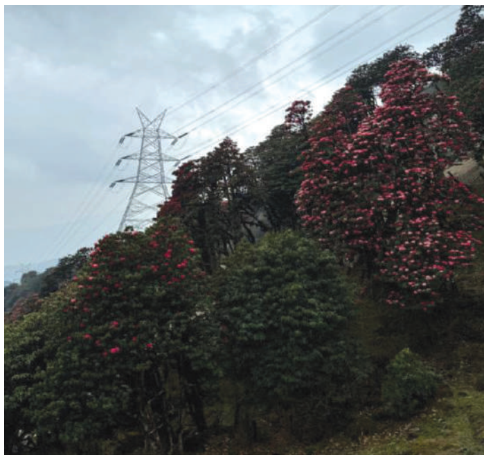
Under KC-4, the Second Circuit Stringing of Basantapur-Dhungesanghu 220 kV line
