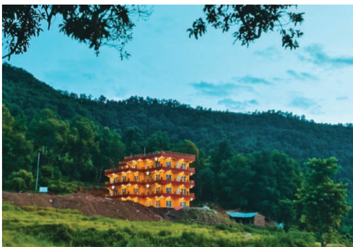
Construction of office building at New Damauli Substation
