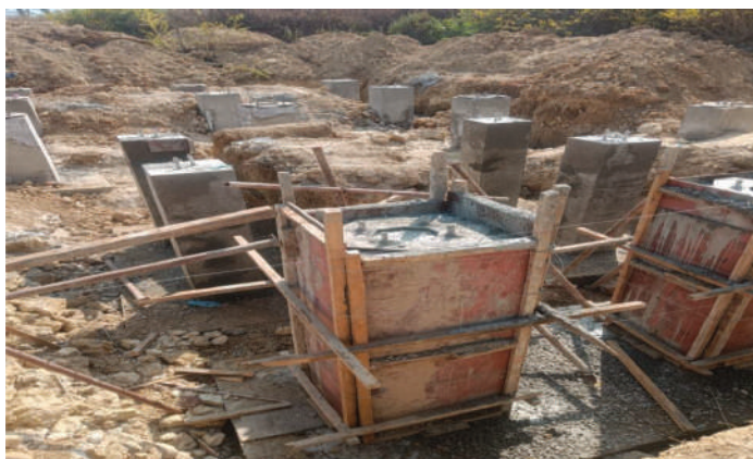
132 kV bay foundation at Matatirtha
