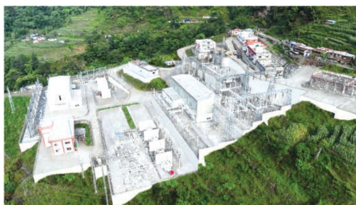
Under Construction Khudi Substation
