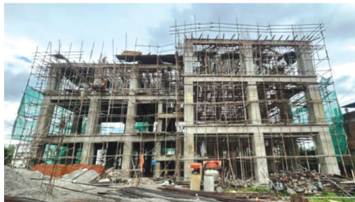
Thimi Control Building cum GIS Hall under Construction
