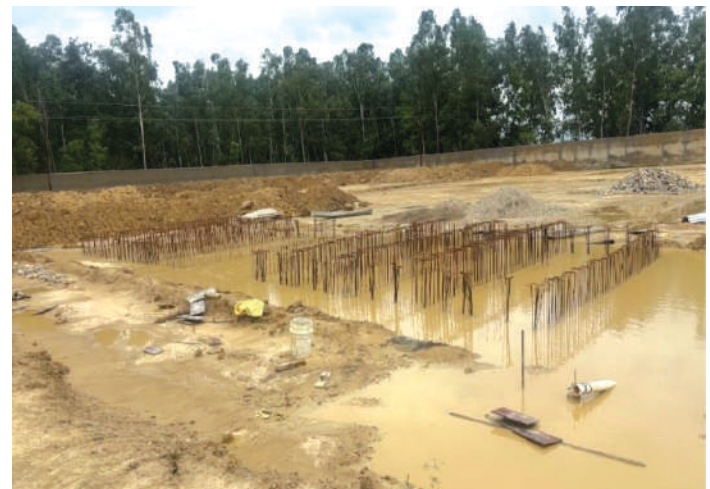
Transformer Foundation Works for 63 MVA Transformer Installation
