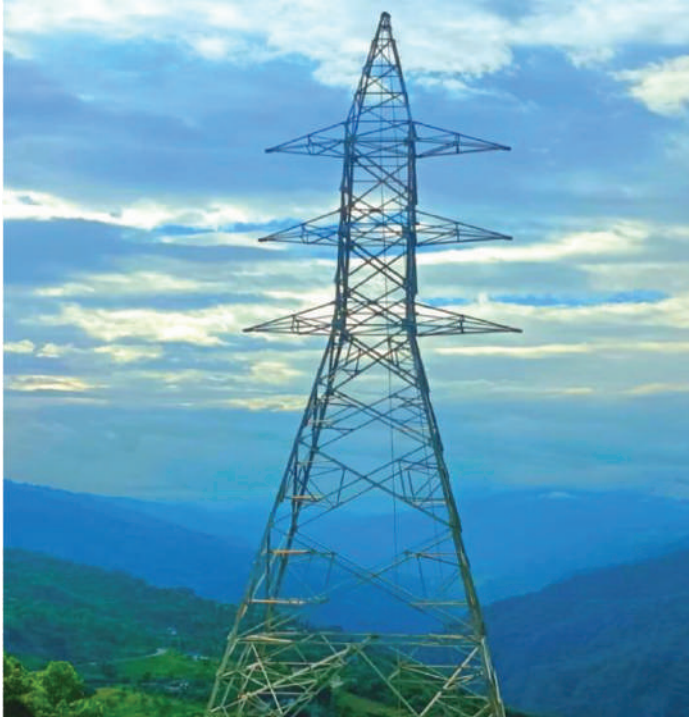
First Erected Tower
