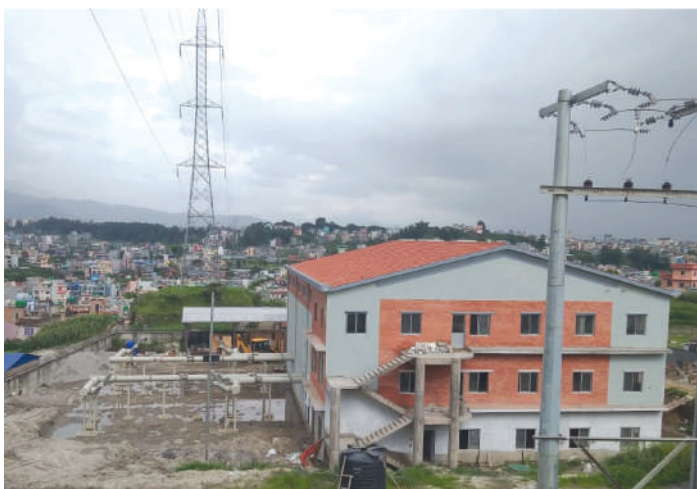
Final stringing at AP 44/0
