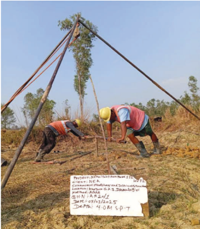
Sub Soil Exploration Works for Tower Foundation
