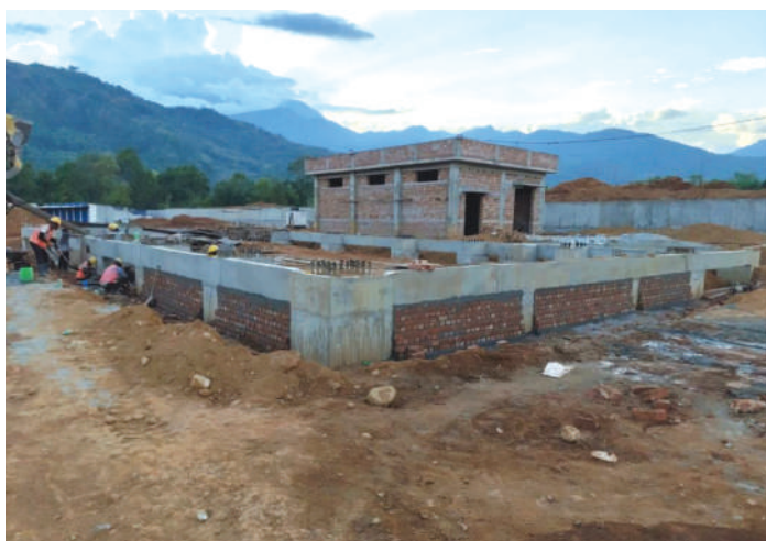
220kV GIS Building Completed upto Plinth Level
