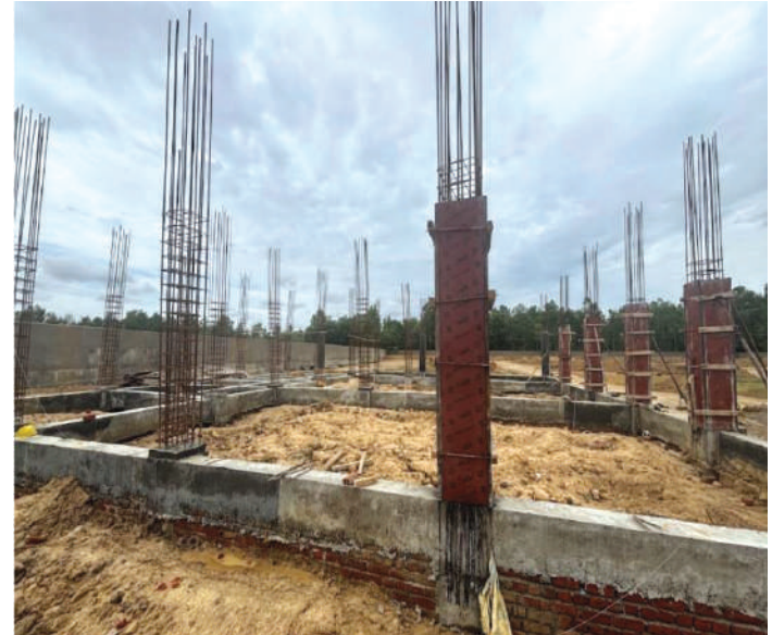
.Control Room Building Under Construction
