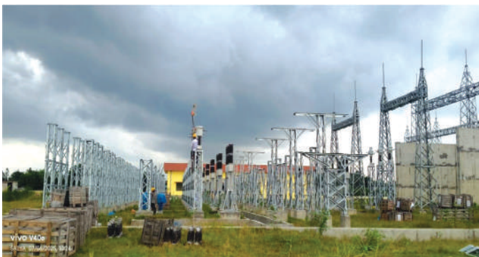
Completion of 33kV equipment support structure for Keraun 132/33kV Substation Work
