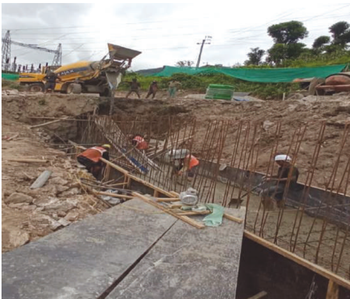
Bay Civil Works at Amarpur S/S
