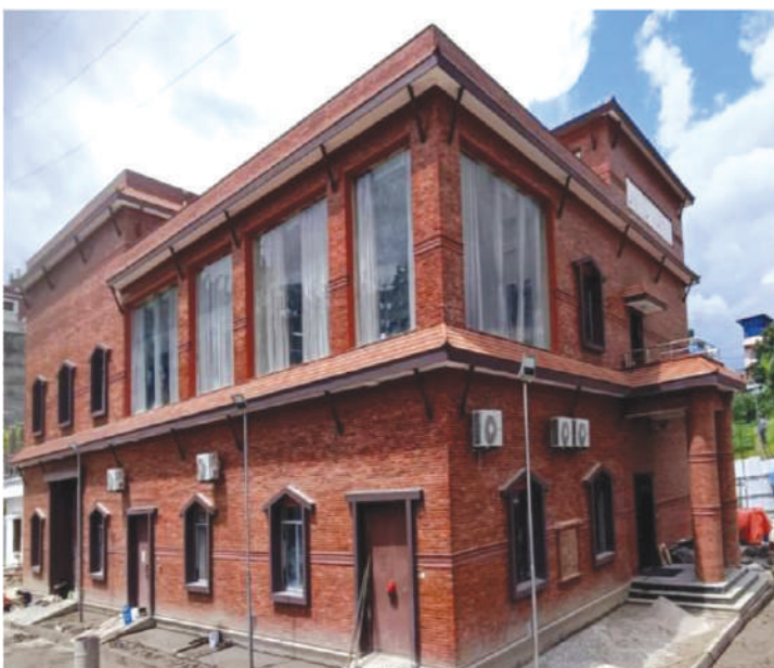
Control Building of Mulpani Substation
