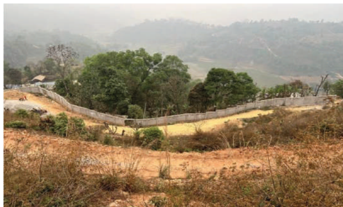
Lapang 220/132/33 kV GIS Substation construction site.
