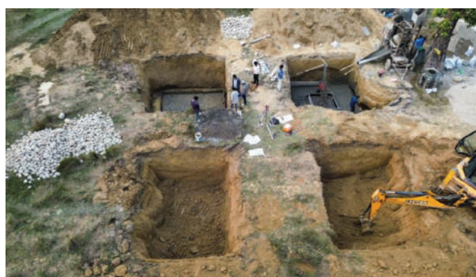
Foundation works for Sunwal-Hakui Transmission Line tower
