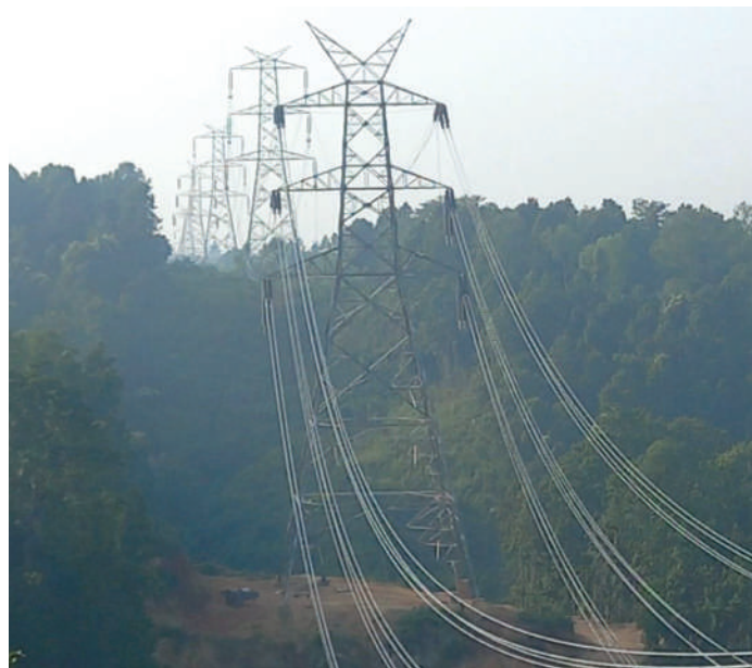
400 kV Double Circuit QUAD ACSR Moose Conductor Stringing work in progress
