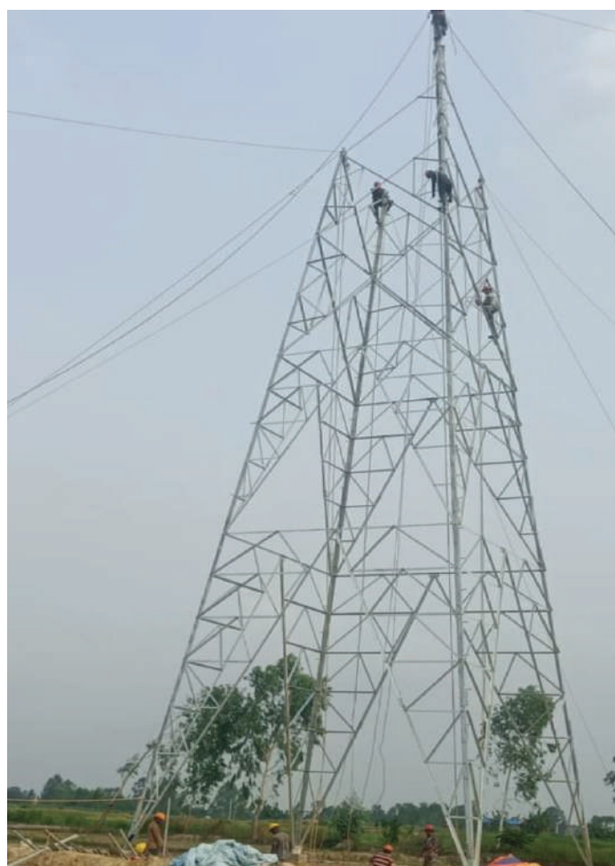
Tower Erection works
