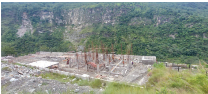
Construction of CR Building and 220kV GIS Building, Rahughat Substation
