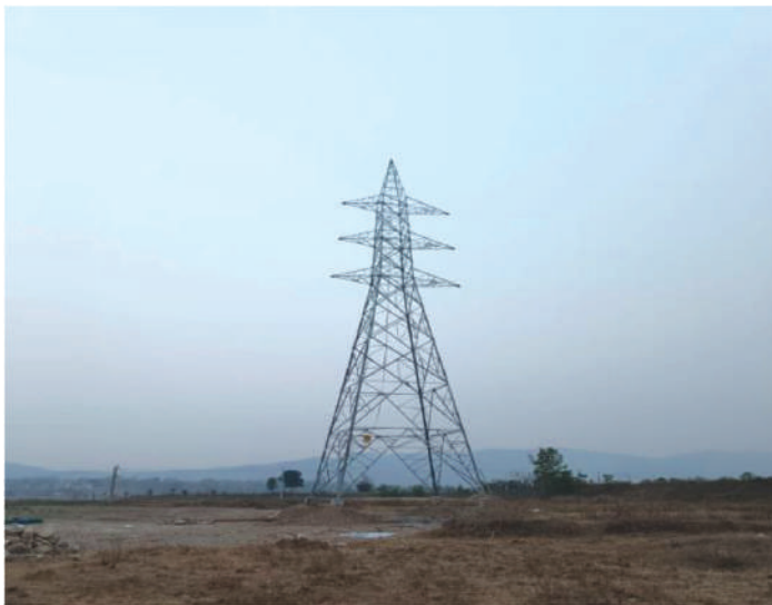
Tower Erection at Dang district
