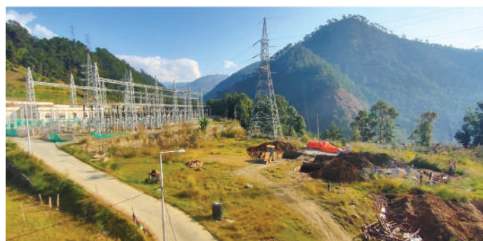
New Modi 132kV Substation (with 2 Bay expansion & Foundation work)
