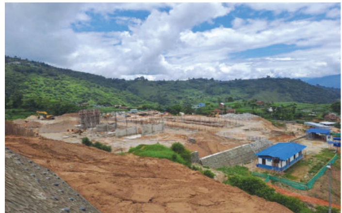
Lapsipedi Substation Site illustrating Transformer and PEB building Foundation Area
