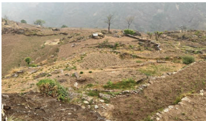
Borang 132/33 kV AIS Substation construction site.
