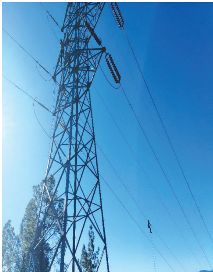
Chameliya-Attaria 132 kV TL Broken Conductor Maintenance Works between T.N. 183-188
