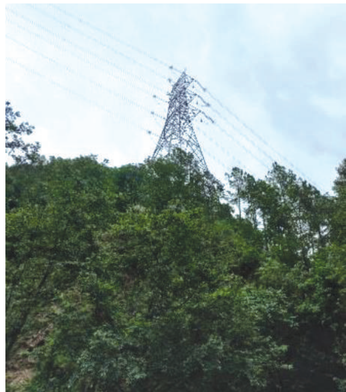
Final stringing at AP 44/0
