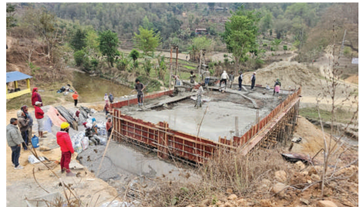
Construction of Bridge over the Chhabdi River
