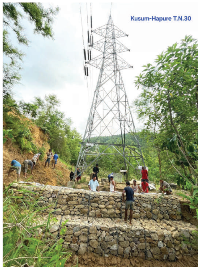
Tower protection works at Hapure-Kusum
